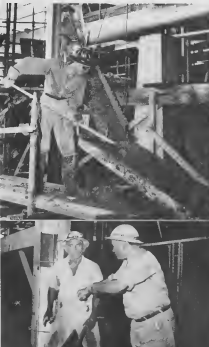
WORKMEN SPREAD approximately forty yards of concrete into the area that will eventually become the foundation for a new turbine in No. 2 Powerhouse. The first pour of concrete formed the mat. There is other pours before the foundation in the Powerhouse pump room is ready for the 7500 KW turbine.
